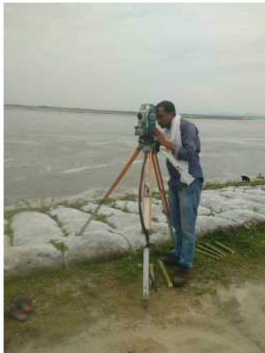
Fig.3.2. Survey work near proposed bridge location
