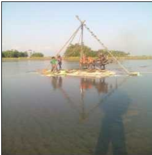
Fig 3.3 c) Boring at Pier -14 (BH-9)
