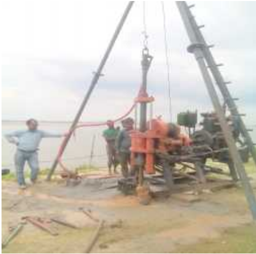
Fig 3.3a) Boring at Right abutment (BH-1)
