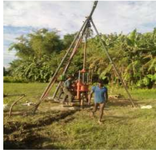
b) Boring at Pier -18 (BH-11)
