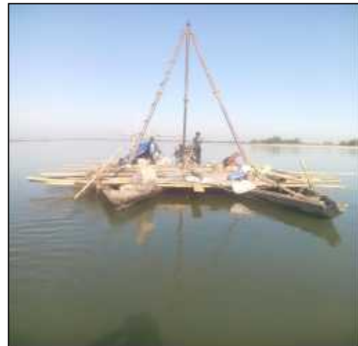
d) Boring at Pier -2 (BH-2)
